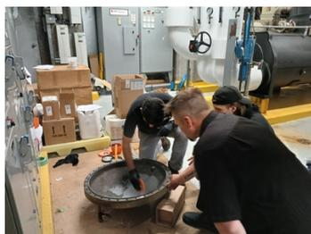
Metal resurfacing with Belzona 1121
