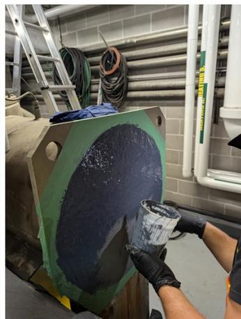
Coating with Belzona 1321
