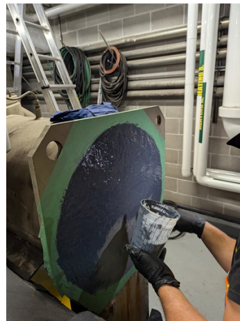
Coating with Belzona 1321
