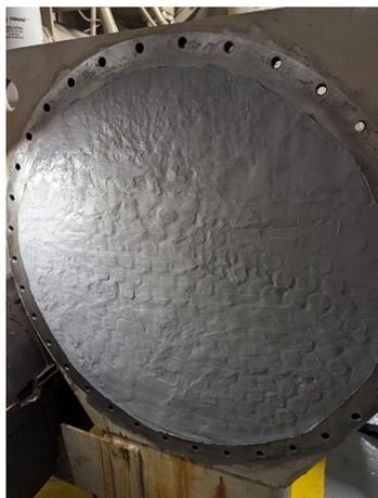
Surface resurfaced with Belzona 1121
