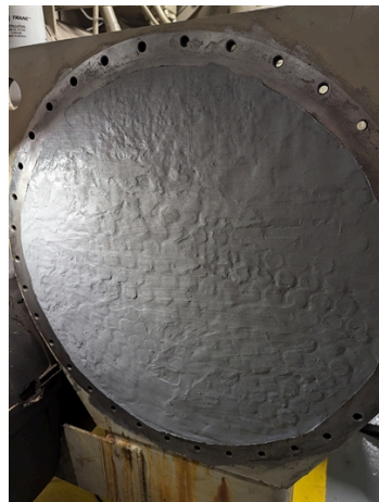
Surface resurfaced with Belzona 1121
