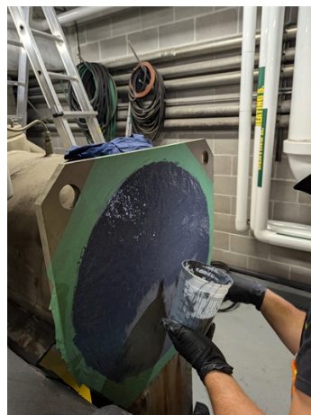
Coating with Belzona 1321
