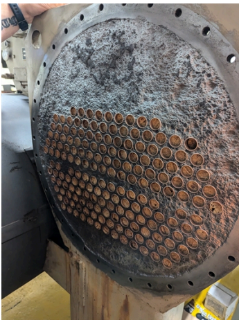
Tube Sheet after surface preparation
