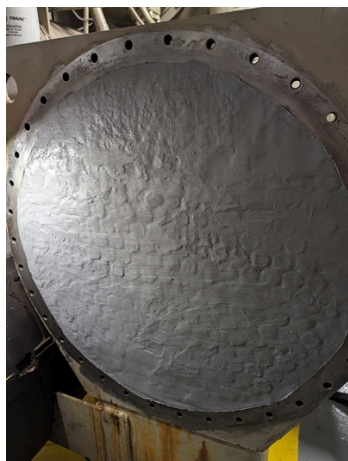
Surface resurfaced with Belzona 1121
