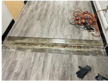
Plate Removed area was cleaned and backer rod was added.
