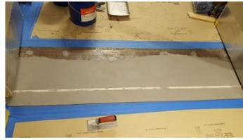
Joint was rebuilt with Belzona 4131, Belzona 2211 was used to form the joint and Belzona 2911 conditioner was used as a primer.
