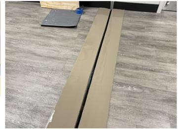
Belzona 5231 was used as the topcoat.
