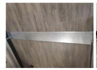
Metal plate was installed when Plate Removed area was hospital was renovated and was a trip hazard.
