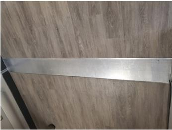
Metal plate was installed when hospital was renovated and was a trip hazard.
