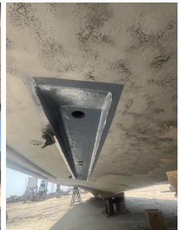
Application of 2nd coat of Belzona 5821 in grey
