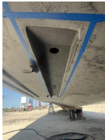
Application of Belzona 1121
