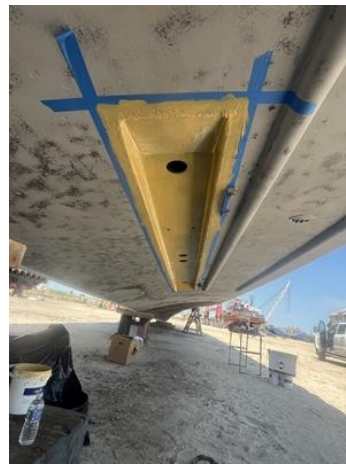
Application of 1st coat of Belzona 5821 in yellow
