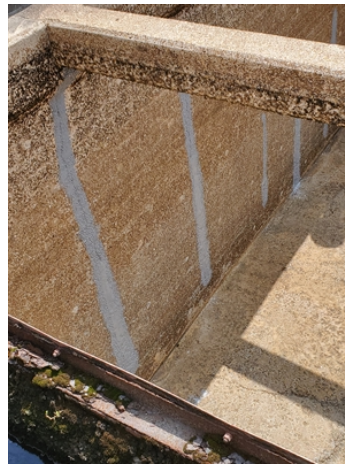
Repair with Belzona 3121
