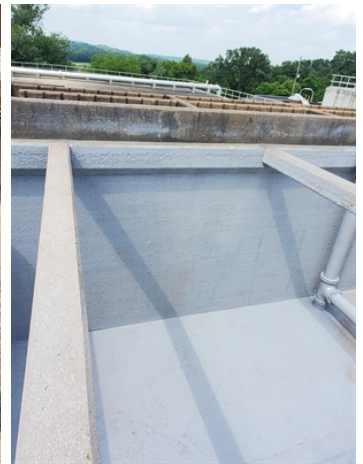
Final application with Belzona 5812DW
