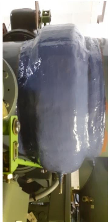
SF6-FIX leak sealing repair completed, with vent pipe left open at 6 o'clock position until full cure is achieved. Vent pipe is capped off following full cure.
