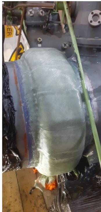
Belzona 7311 applied to repair area incorporating Belzona 9341. 5x layers of Belzona 9371 using Belzona 1981 resin for wetting.
