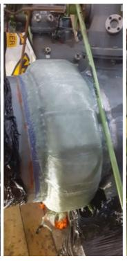
Repair area substrate prepared Belzona 7311 applied to repair area incorporating Belzona 9341.
