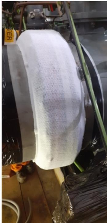
Repair area substrate prepared utilising bristle blaster and breather membrane installed.
