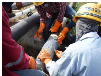
Wetting out substrate with Belzona 1111 after Surface Prep and Solvent Cleaning
