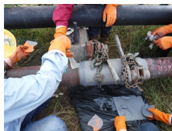
Plate Bonding with Belzona 1111
