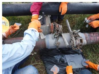
Plate Bonding with Belzona 1111
