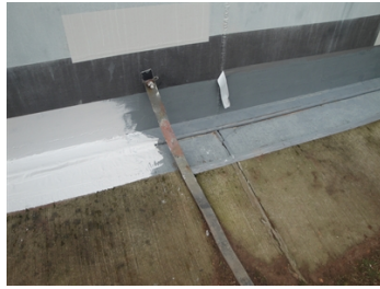
Belzona 3921 applied & 1st coat of Belzona 3131
