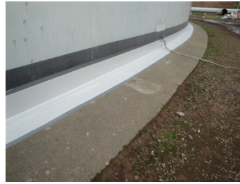
1st coat of Belzona 3131
