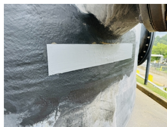
After: We applied 1 coat of Belzona 1111 with Reinforcement Cloth Engrained.
