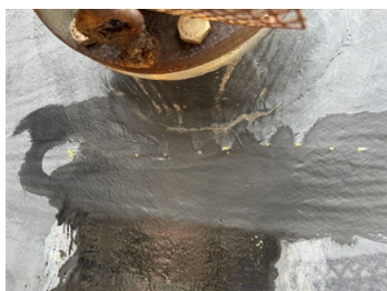
Before: Yellow Dots mark the crack, we cleaned the area with Acetone
