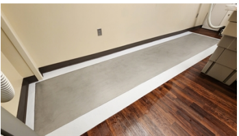
Transitions formed from steel plate to laminate with wall cove base reinstalled
