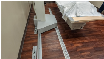
X-ray machine's weight is visibly not supported properly causing bowing of the floor underneath
