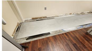
Steel plate cold bonded to concrete
