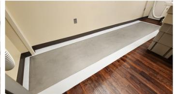
Transitions formed from steel plate to laminate with wall cove base reinstalled
