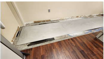
Steel plate cold bonded to concrete
