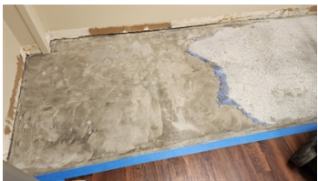
Flooring was removed to reveal uneven substrate
