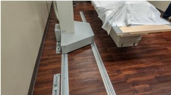
X-ray machine's weight is visibly not supported properly causing bowing of the floor underneath
