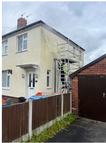
Preparation: Washing down the rendered walls with HP water & fungicidal wash prior to fixing any cracks or damaged rendered surfaces
