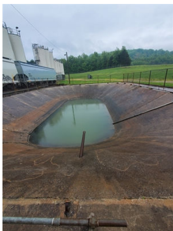
Containment area before restoration.
