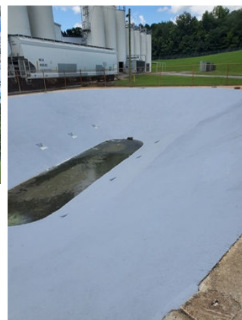
Containment area finished with two coats of Belzona 5231
