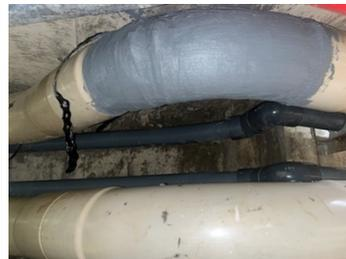
Full application and reinforced wrap using Belzona 1161 and Belzona 9341 Done in August 2023
