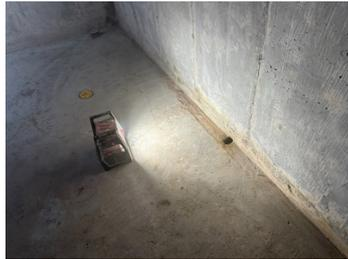
Hole located. A section of wood formwork was at grade and had deteriorated allowing the reservoir to lose a significant amount of water daily.
