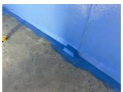
Hole sealed and 1st coat of Belzona 5812DW was applied.
