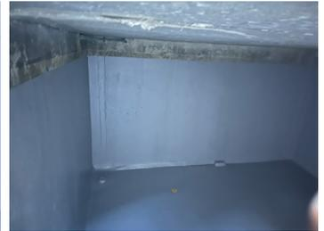
Completed 2 coats with Belzona 5812DW.
