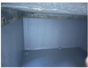
Completed 2 coats with Belzona 5812DW.
