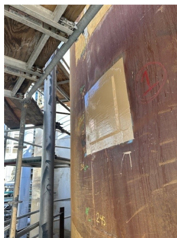
Close-up of finished application of plate bonding.
