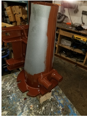
Surface prepping the asset.
