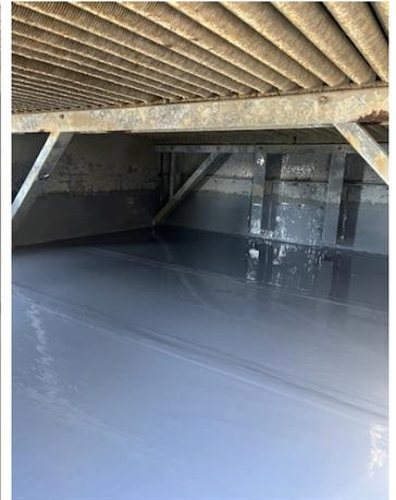
Second coat of Belzona 5815 grey.
