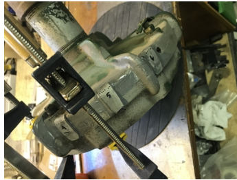
Shows pump having had Belzona 1212 applied to the ground crack and 6 steel tabs bonded around the crack.
