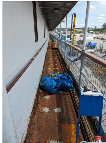
Entire deck after weeks of application,
