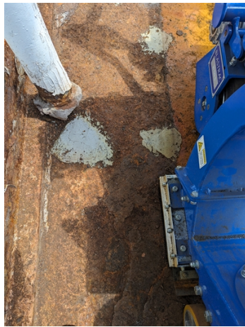
Deck after application of Belzona 1111
