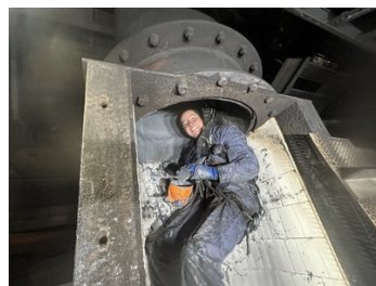
During application of Belzona 1321.
