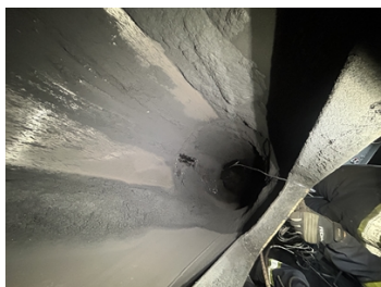
Chute prior to surface preparation.
