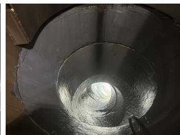
Completed application with Belzona 1321.
