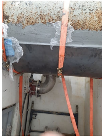
Plate bonding over the most critical area.
