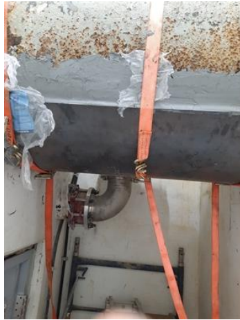
Plate bonding over the most critical area.
