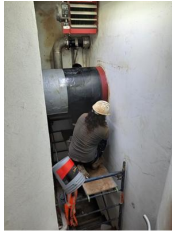
Applying SuperWrapII to strengthen the entire pipe section.
