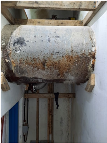
Defective pipe in need of reinforcement.
