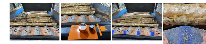
Steel grit blasted at welds that Belzona 1818 ready to be used. Belzona 1818 applied. would frequently wear away.
