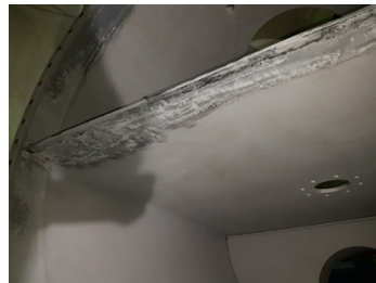
Repaired divider bar
