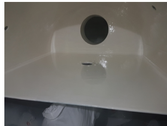
Full coat of Belzona 1331 being applied
