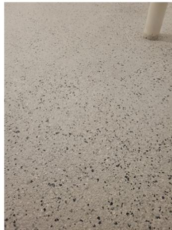
Vinyl flakes applied onto Belzona 5231.
