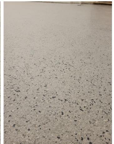
Belzona 5233 was applied as the clearcoat topcoat.
