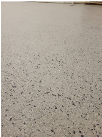
Belzona 5233 was applied as the clearcoat topcoat.
