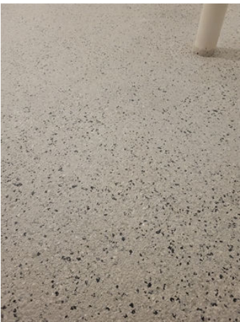
Vinyl flakes applied onto Belzona 5231.
