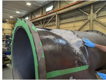
Belzona 4141 application to make a uniform shape.
