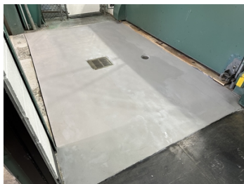
Completed application, 14 buckets of Belzona 4111 Magma Quartz were used to complete the restoration
