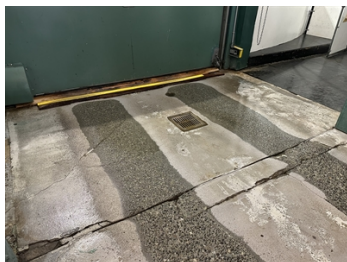
Condition of concrete where the Zamboni exits the ice-sheet
