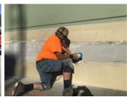
After patching the area using Belzona 4111 magma quartz an was left for the painting crew angle grinder and sanding disc to repaint. were used to achieve smoothness and a good transition between the old and new coating.
