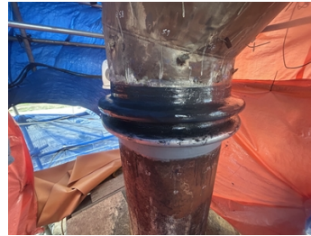
Belzona elastomer and cloth applied
