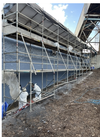
Application of Belzona 4111 to repair concrete.
