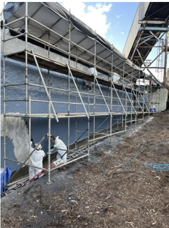
Application of Belzona 4111 to repair concrete.
