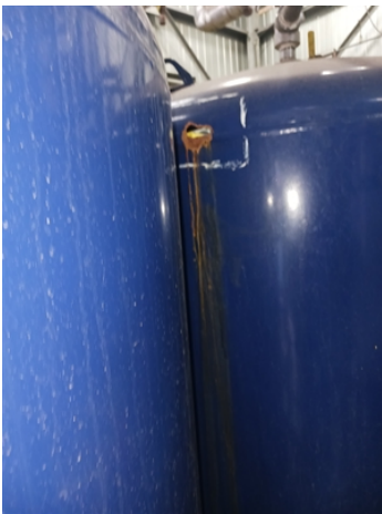
Tank showing hole defect.
