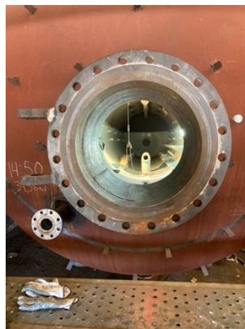
application in progress
