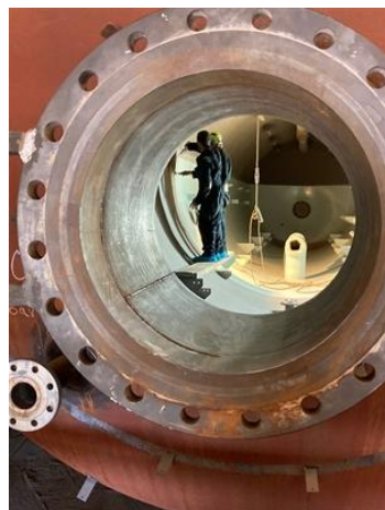
application in progress
