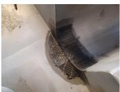
Damages in the gutter were detected with a test spray.
