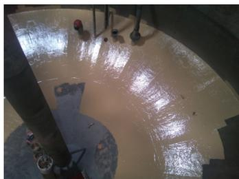
Application of the product Belzona 5811 (Immersion Grade) in the first layer.
