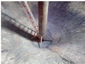
Damaged tank bottom
