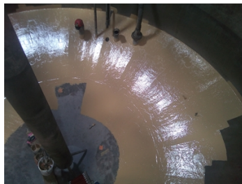
Application of the product Belzona 5811 (Immersion Grade) in the first layer.
