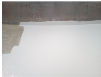
Application of the product Belzona 5811 (Immersion Grade) in the second layer.
