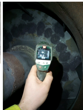
Since the repair was carried out in the winter, the fan had to be heated and the temperature had to be controlled.
