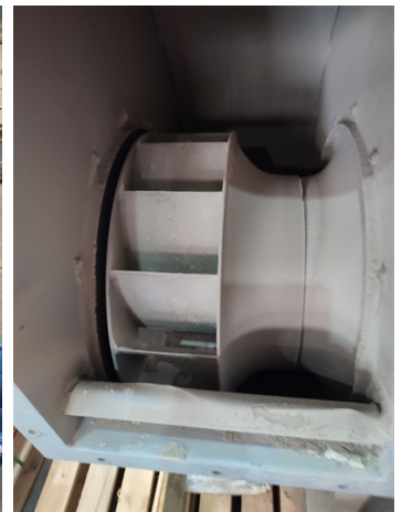
Fan wheel before repair
