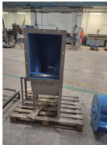
Application of the product Belzona 1341 on the fan box
