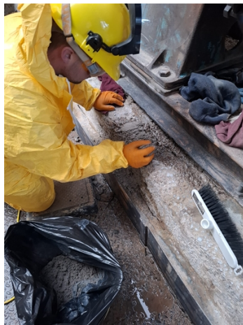
Application of Belzona 4131
