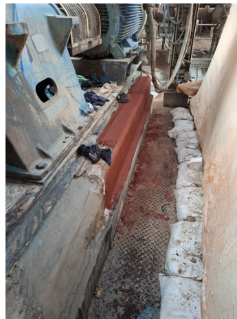
Application of Belzona 4181
