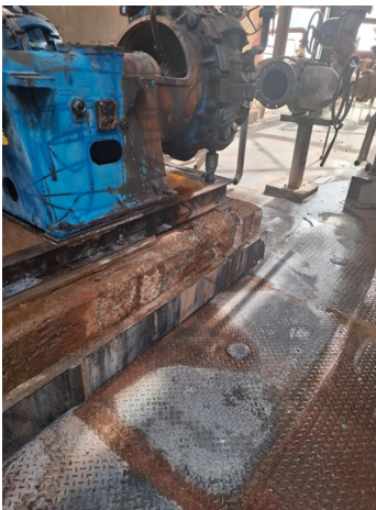
Initial condition of plinth
