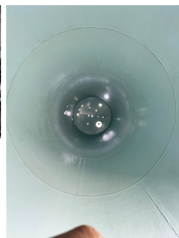
Final phase with Belzona 1593
