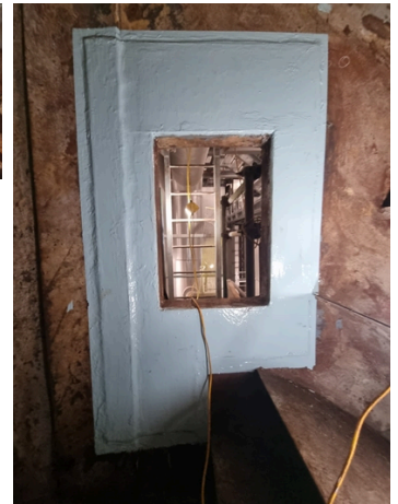
Plate bonding and coating of localised defect.
