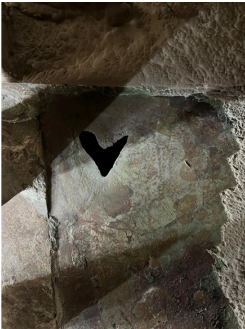
Internal through hole defect.
