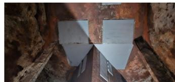
Plate bonding and coating of localised defects.
