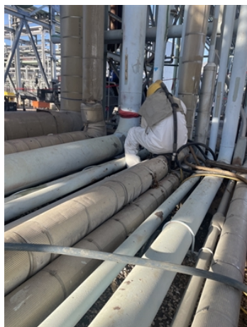
Application of Belzona 1161.
