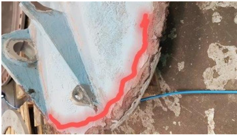
Worn out metal
