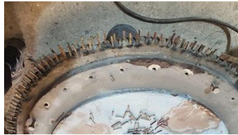
Welding metal supports before applying Belzona 1111 (Super Metal)
