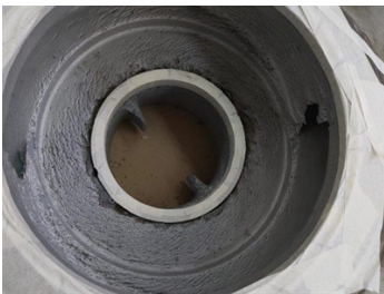
Erosion evidence on pump component due to high solid content
