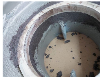
Pump surface was rebuilt with Belzona 1311 (Ceramic R-Metal)
