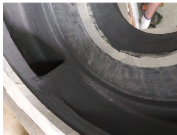
Surface preparation on the pump before the application of Belzona system
