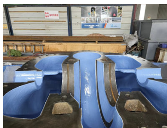
2 coatings of Belzona 1341 completed
