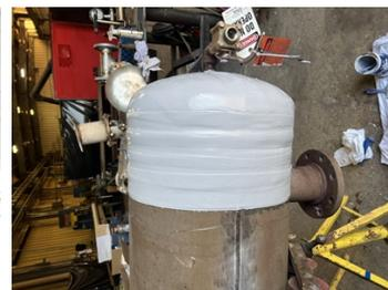
Surface preparation of areas of repair, all identified cracks terminated as per system leaflet TCC-1
