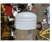
repair, all identified cracks terminated as per system leaflet TCC-1
