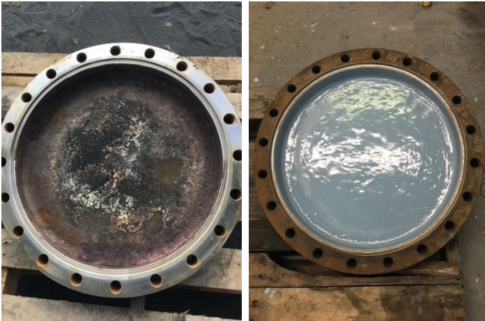
Cooling Water Head Before
