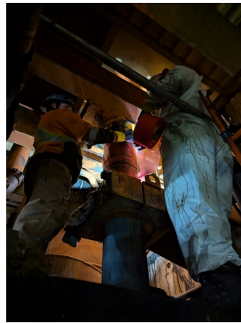
Super Wrap II was installed.
