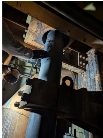
Pipe and metal plate covered with Belzona 1212.
