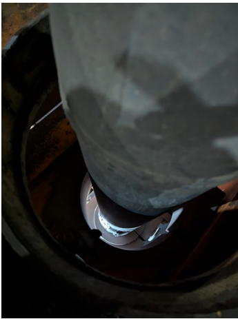
Pipe after surface preparation.
