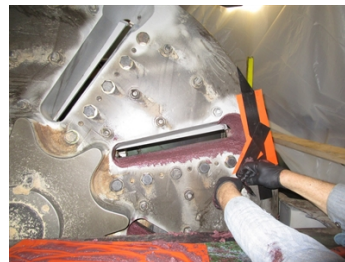
Belzona 1811 applied with some mixing board pieces taped in place to help with the profile.
