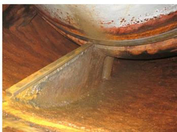
Initial inspection, after use of a wire wheel to see the corrosion damage.
