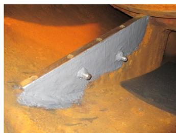
Belzona 1311 applied to the corroded areas and over coated with Belzona 1321.
