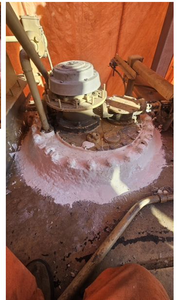
After application of Belzona 5831LT
