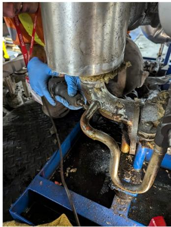
Sealing with Belzona 1221.
