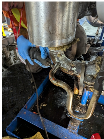
Sealing with Belzona 1221.
