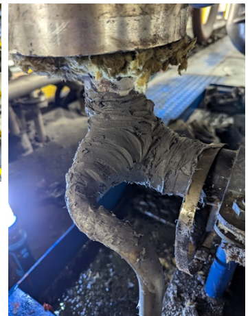
Entire area covered with Belzona 1511.
