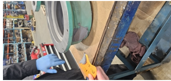
Rebuilt with Belzona 1111.
